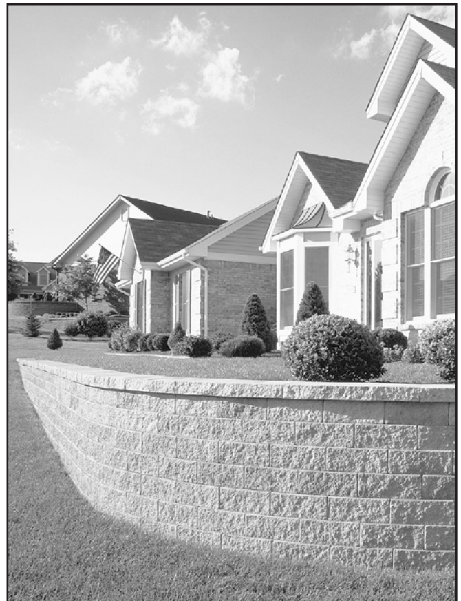
Careful base course planning for convex curves is important when building tight curves.
