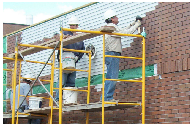
Photo 3 Installation of Modular Panel
